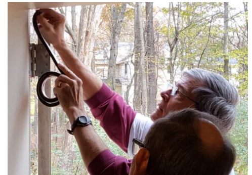
Apply weather stripping around doors.
